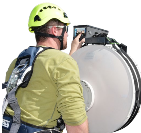
Antenna Alignment Process
